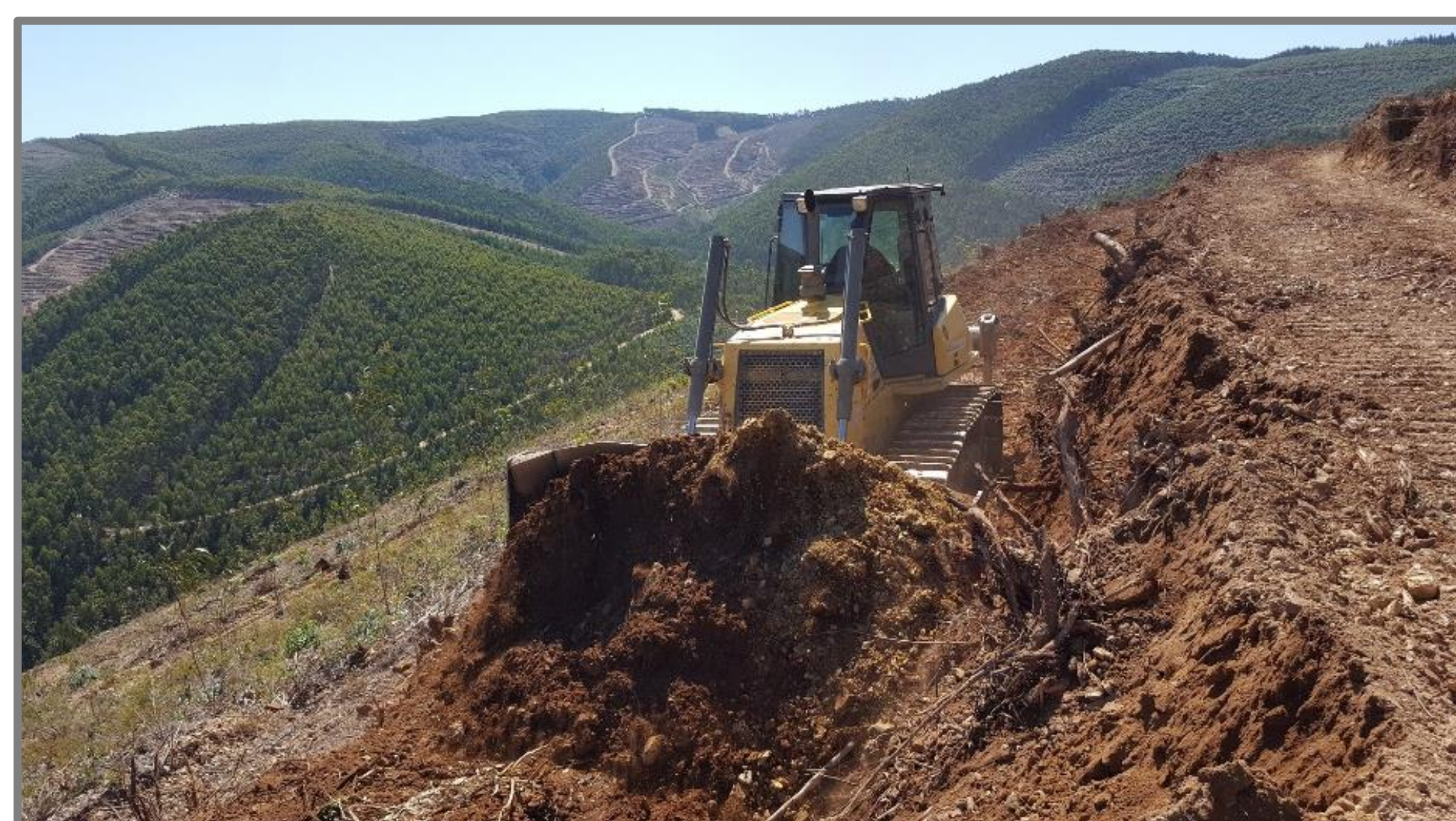
Figure 1 – Terraces being built by a bulldozer in July 2019 near the village of Boialvo (Anadia Municipality).
