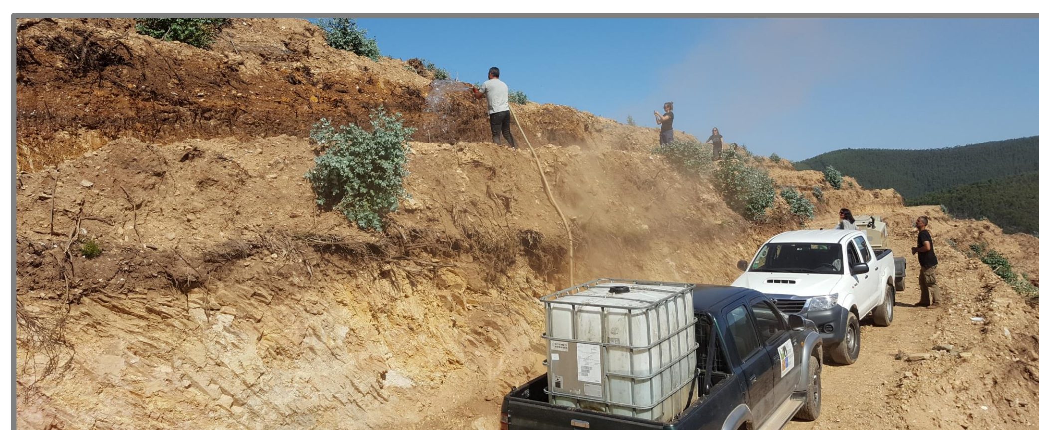
Figure 3 – Application of synthetic polyacrylamide by spraying the mixture using a hydroseeder.
