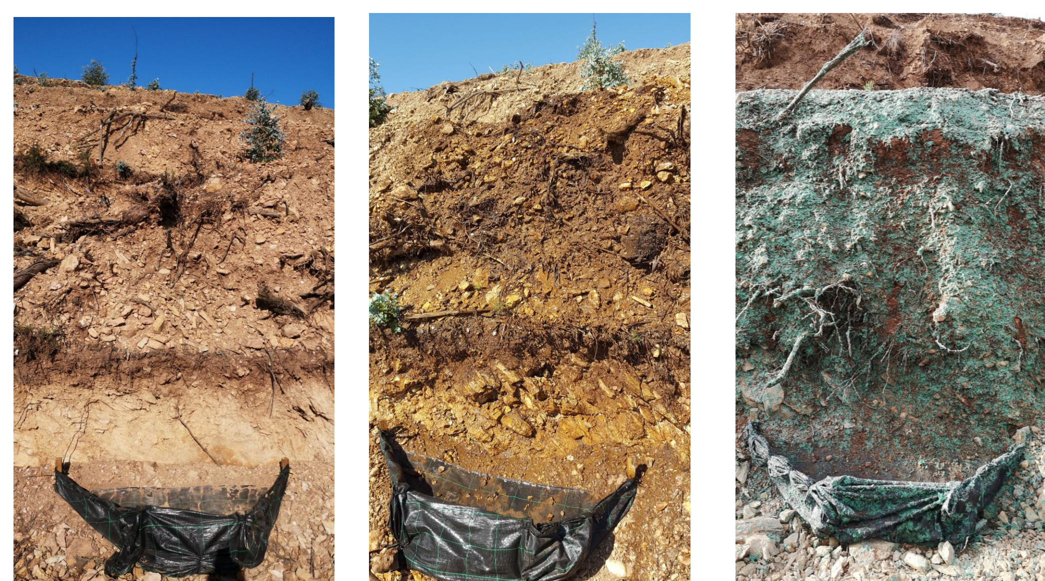
Figure 2 – Sediment traps installed in the bottom of the terrace wall (1) control (2) application of polyacrylamide (3) application of hydromulch.
